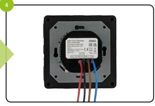
Connect the thermostat according to the wiring diagram.
