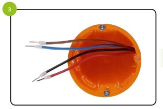
Make sure that the wires are not under 230V AC.
